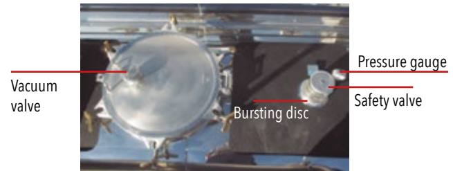
FIGURE 37: Vacuum valve + safety valve + bursting disc
