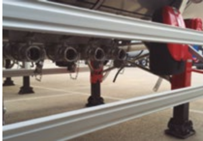
FIGURE 30: Individual piping outlets at side
