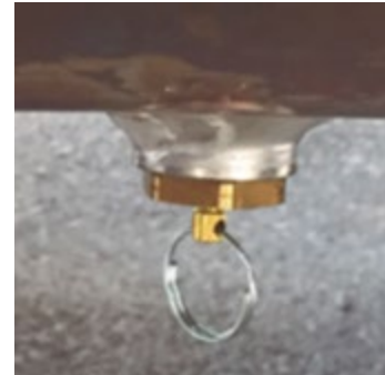
FIGURE 9: Manual purge system
