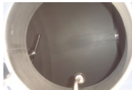
FIGURE 23: Inner cleaning shower with overflow sensor
