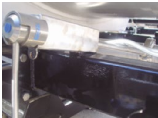
FIGURE 28: Manual valve with handle extension to be operated from one side
