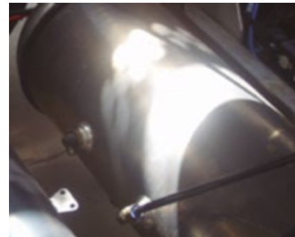
FIGURE 10: Automatic purge system
